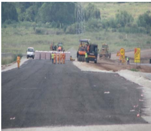
Voortrekker Road – Phase 1 under construction
